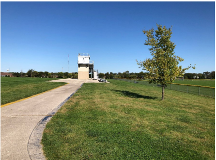
Athletic Field with Concessions & Toilet Rooms
