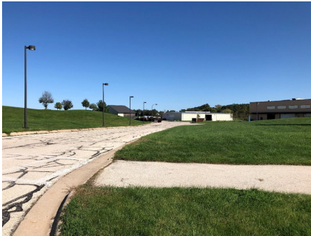
Support Service Buildings
